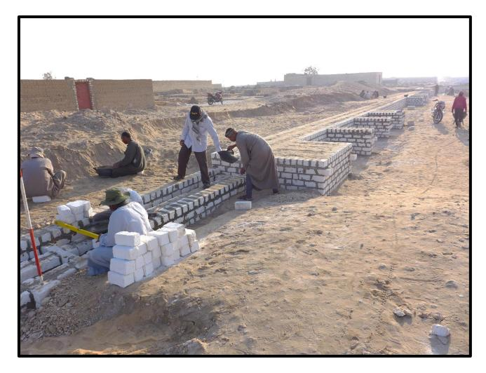
Figure 3: View of the same area as Figure 2 but viewed to the north-east and after the new stone foundations had been nearly finished. The thick projections added to the main wall represent the beginnings of walls which cross the temple from side to side. When the intended scheme is finished, none of the small blocks will be visible.
