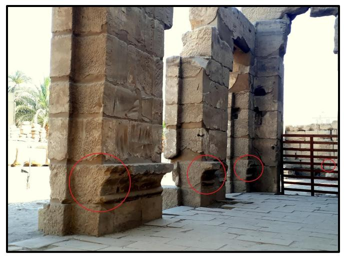
**Figure 9**: Luxor temple, part of the preserved façades of three of the small rooms on the south-east side. The red circles indicate parts of the cavetto cornice which originally ran continuously and fronted the raised floors inside each room. Floors and partition walls were removed in later times. The smallest of the red circles is the location of Figure 8. Photograph by Juan Friedrichs.
